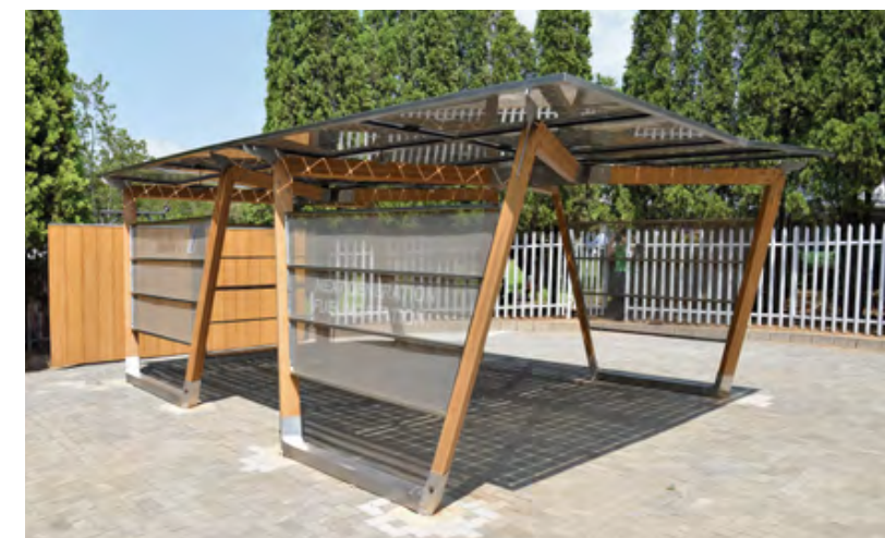
Car port in South Africa: charging electric vehicles with solar energy.
